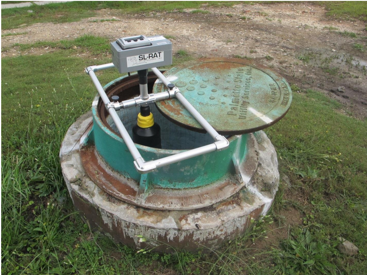
Figure 2. SL-RAT Transmitter Unit Deployed on a Manhole
