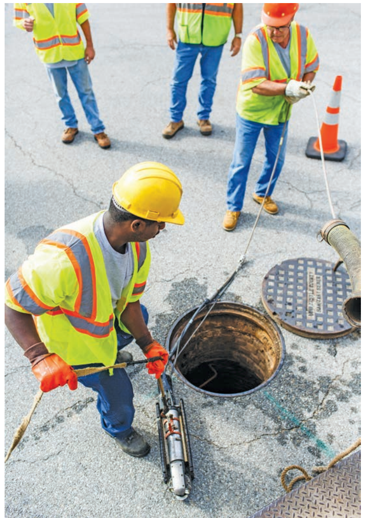
Top left: Al Toto monitors water pressure and flow from a Vector jetting truck while flushing a sewer main. Above: Camera operators Kwamane Finch (left) and Gary Guillotte prepare to send a camera down to inspect a sewer line.
