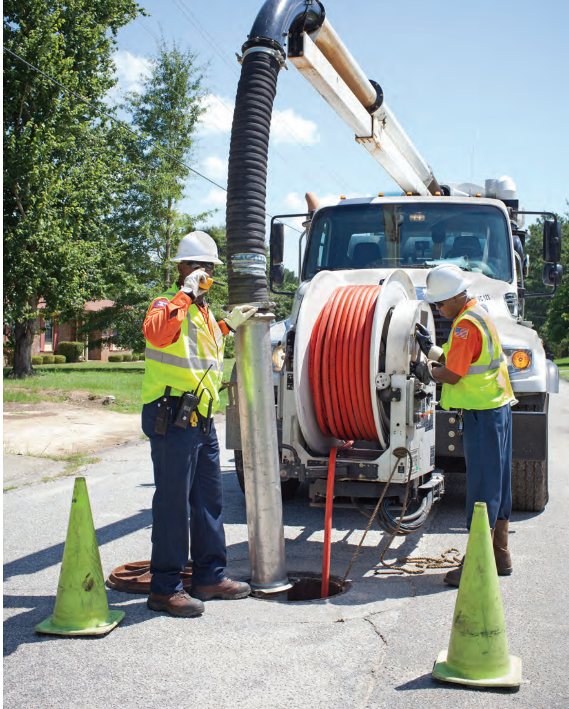
Nathan Rothwell, left, and Frank Minglehoff clean out a section of pipe with the Vector 2100 Series vac truck.
